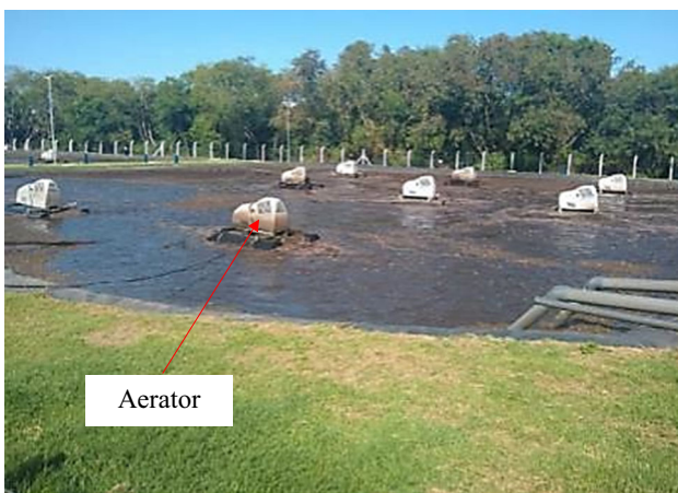
Fig. 1 Effluent treatment pond where aerators/mixers are used
