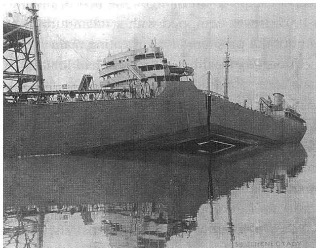
Fig. 1 Liberty ship Schenectady in the Portland shipyard split in two while still under construction in 1943
