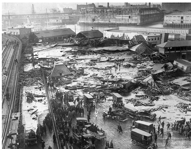
Fig. 2 Boston Molasses tank failure wrecked an entire neighborhood in January 1919
