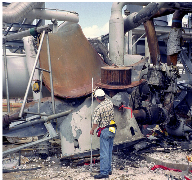
Fig. 3 Brittle fracture of a pressure vessel is sudden and catastrophic, resulting in loss of containment of product and energetic fragmentation
