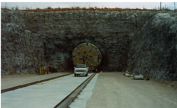
Fig. 3—Face of tunnel boring machine exiting Yucca Mountain after construction of the initial tunnel, which is known as the Exploratory Studies Facility. The SAM materials are an option for the disk cutters for tunnel boring machines that will be required to excavate the 65 km of 5-m-diameter emplacement drifts at Yucca Mountain.
