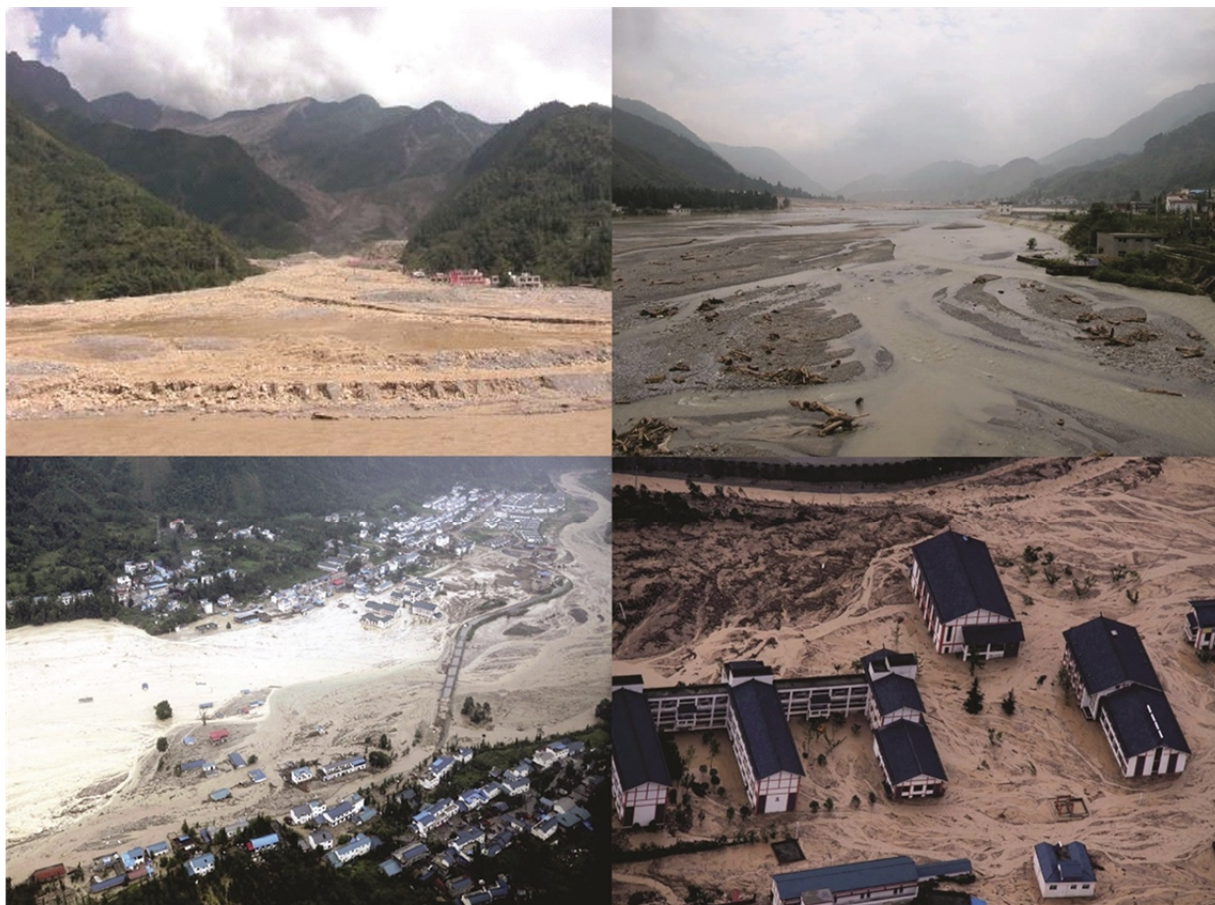
Fig. 1 On August 12 - 14, 2010, a series of rainfall-induced debris flows occurred in 21 ravines around the towns of Qingping, Mianzhu City, Southwest China's Sichuan province, in areas previously affected by the 2008 Wenchuan earthquake. Consequences were devastating particularly in the housing and infrastructure sector (top right photo by courtesy of Hong Xie, other photos by courtesy of Yong You).
