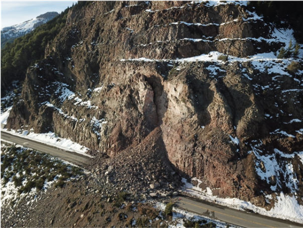
Fig. 10 Rockfall blocking the access between Villa La Angostura and Bariloche for almost a month, during winter 2019. Photo courtesy of Carlos Tavalla.
