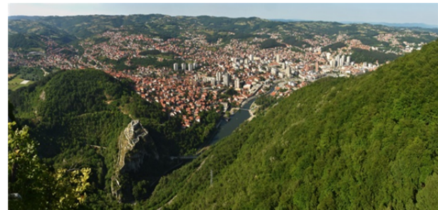
Figure 3 Panorama photo of Užice town with Djetinja River. The town is located just at the lithological boundary. In the foreground, the edge of the limestone plateau can be seen and the ruins of the Medieval fortress are also on a limestone block. In the background, the hilly landscape dissected by fluvial valleys on Palaeozoic metamorphic rocks can be observed.
