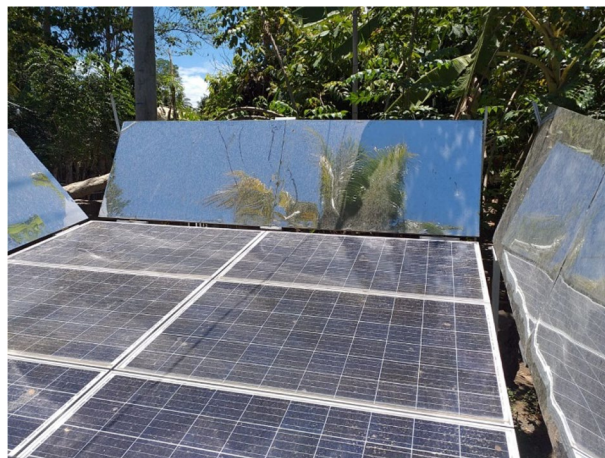
Fig. 6 Sun reflector add-ons to the North Lombok facility resulting from continuous feedback for improvement (source: author's collection)
