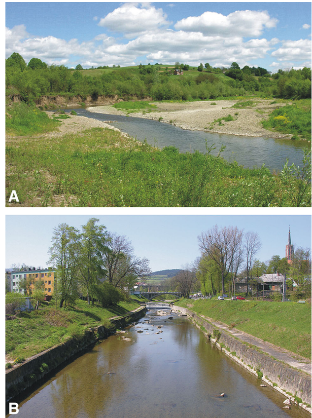
Fig. 2 Examples of near-natural (a) and extremely modified conditions (b) for lateral connectivity of the river ecosystem and channel migration. The unmanaged, sinuous channel can freely migrate on the floodplain. The mode of river channelization presented in the lower photo results not only in the lateral stability of the channel but also in the loss of lateral connectivity of the river ecosystem
