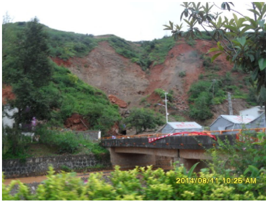
Fig. 8 A small landslides blocked the bridge on the road to the Longtoushan Town
