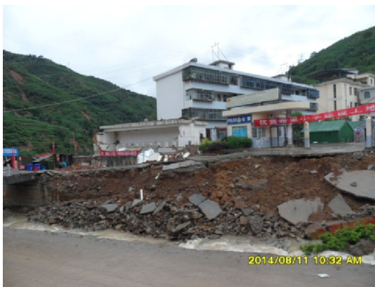
Fig. 9 Collapse of the river bank in Longtoushan Town
