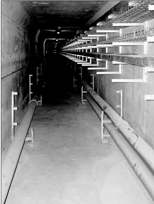
Figure 1 Photo of an existing utility tunnel.
