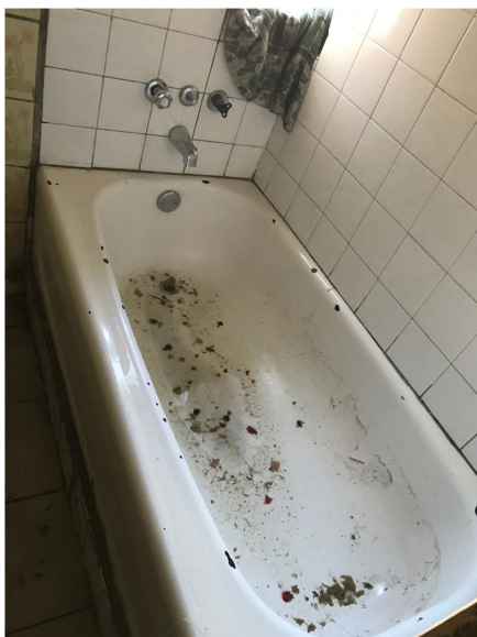
Fig. 1 Plugged bathtub at SRO #1
