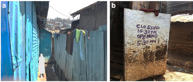
Fig. 7 a Informal formation of slum residential enclaves by fencing and (b) gate in the slum showing agreed opening and closing time
