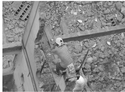
Fig. 7 Manual demolition of reinforced concrete structure in Manila
