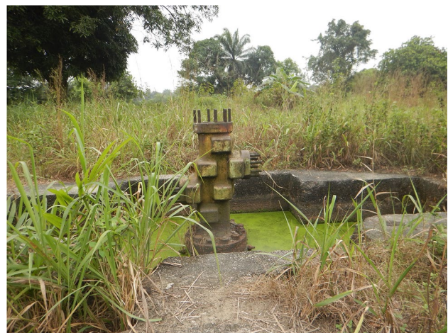
Fig. 6 A well-head near residential area in Gokana local government council
