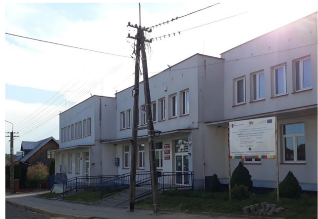
Fig. 1 Analyzed office building (photo by D.A.Krawczyk)
