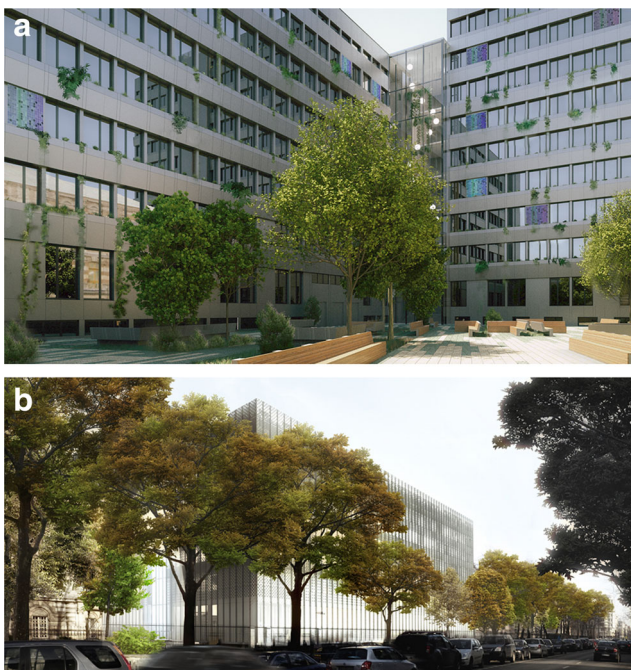
Fig. 10 Faculty of Building Services, Hydro and Environmental Engineering—proposition of the “new skin” screening mechanical areas. BP phase (KODnZEB 2015–2017)
