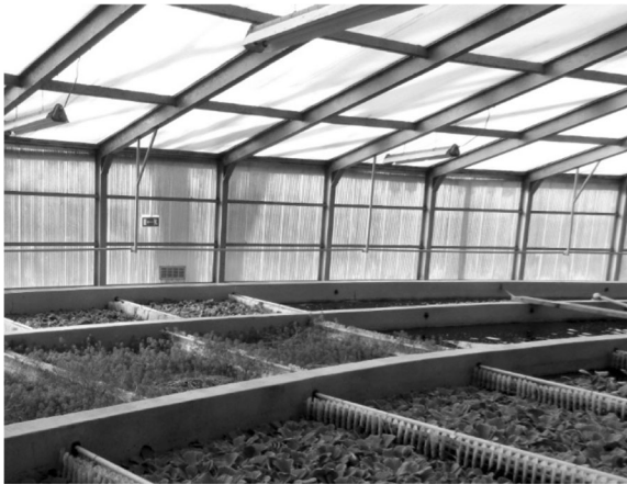
Fig. 2 Hydroponic lagoon located under the roof made of polycarbonate sheets [fot. A. Bawiec]
