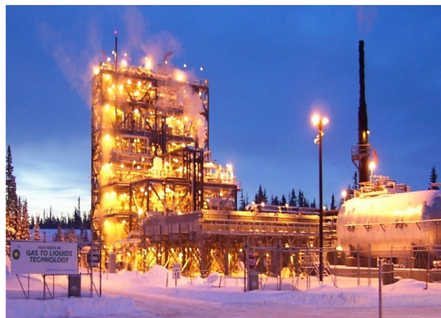
Fig. 3 The Nikiski Demonstration Plant in Alaska, which produced 300bbl/day of synthetic fuels product
