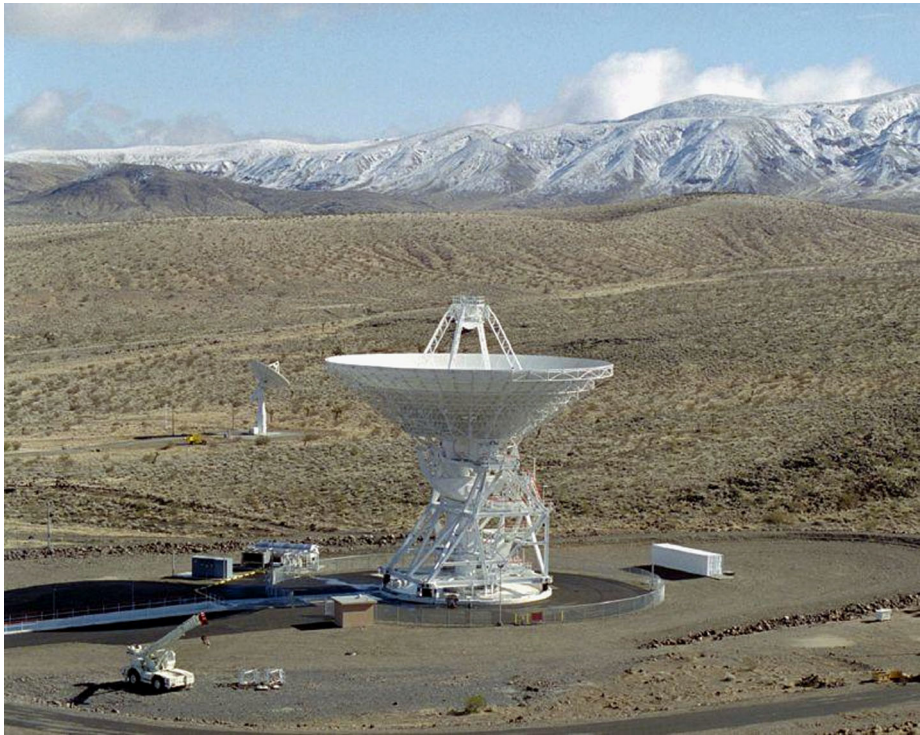
Fig. 3 NASA/JPL Deep Space station 25 (DSS25), a 34-m beam waveguide antenna, shown here in the stowed position. It was specifically instrumented for Cassini radio science with high-stability electronics, Ka-band up-and downlinks, and advanced media calibration systems to correct for tropospheric scintillation (credit; NASA-DSN)
