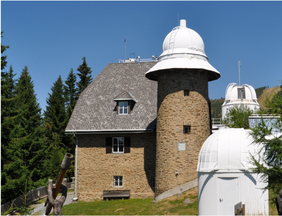
Figure 1 Kanzelhöhe Observatory today. The heliostat was installed in the southern tower (leftmost), in the northern tower (open dome in background) a small telescope for testing purposes replaced the coronagraph after 1948. Since 1973 all observations are performed in the northern tower.
