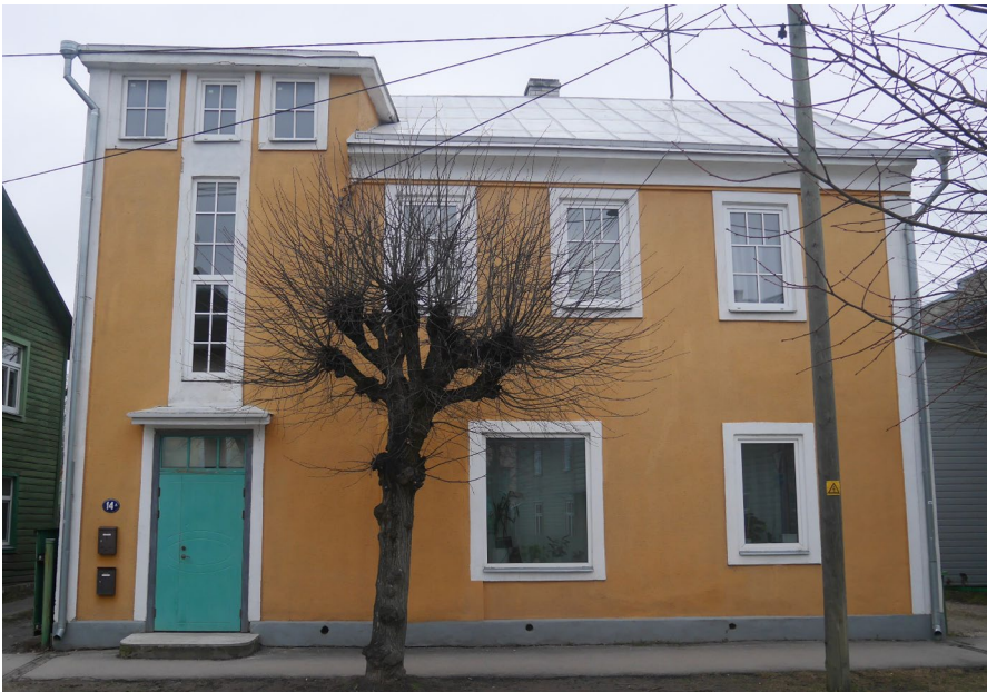
An historical building's facade in Karlova area has been altered with plastic windows and a modern front door
