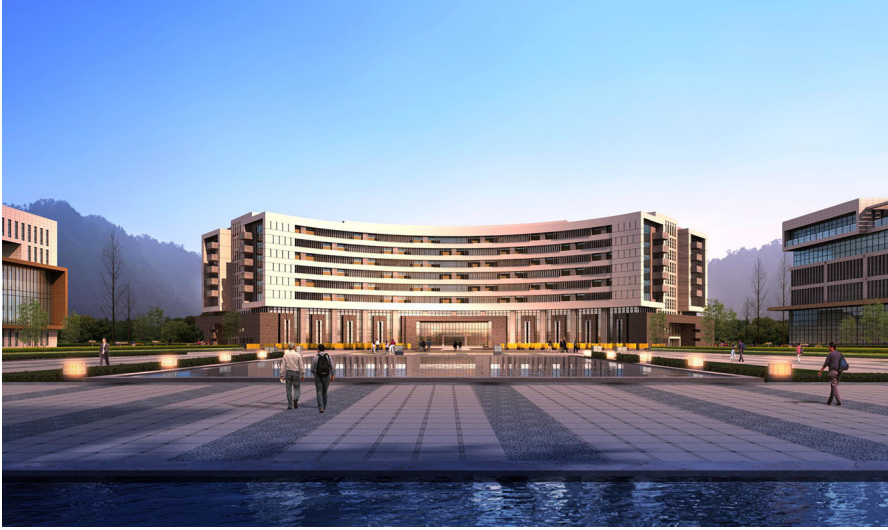
Building of Research Institute of Photocatalysis which occupies 3rd and 4th floors.
