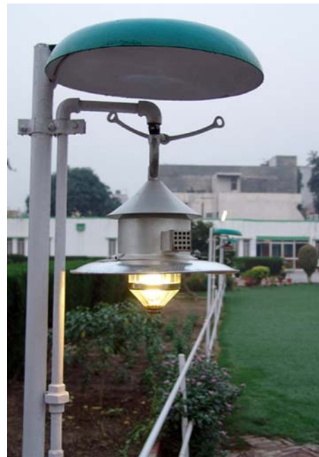
Fig. 3 Lamp powered by local biogas
