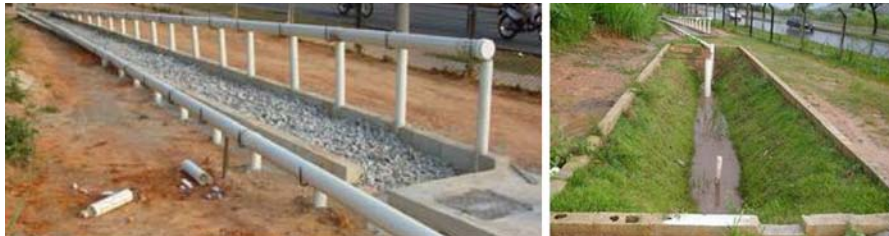
Fig. 2 Infiltration trench ( left ); detention trench ( right )
