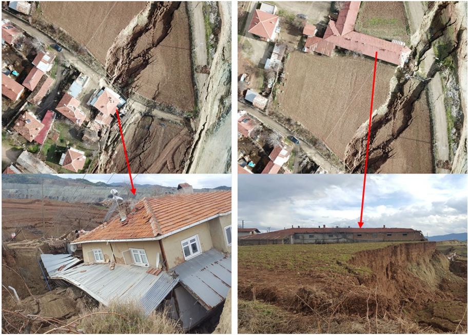
Fig. 2 UAV images and photos: (left) landslide cracks and destroyed building, (right) damaged poultry house
