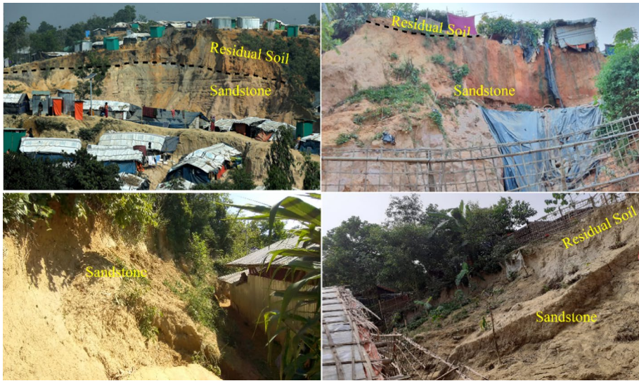
Fig. 2 Landslides in the Kutupalong Rohingya camp
