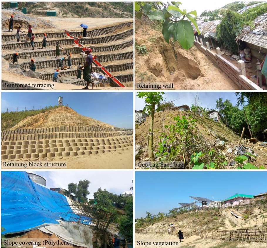
Fig. 6 Different landslide mitigation measures implemented in the KRC area
