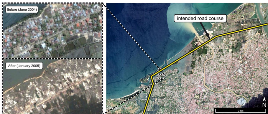
Fig. 6 Intended course of the elevated road in Banda Aceh. Left: Consequences of the 2004 IOT in Banda Aceh (Satellite data composite from Maxar Technologies accessed through Google Earth Pro, vers. 7.3.4.8248)
