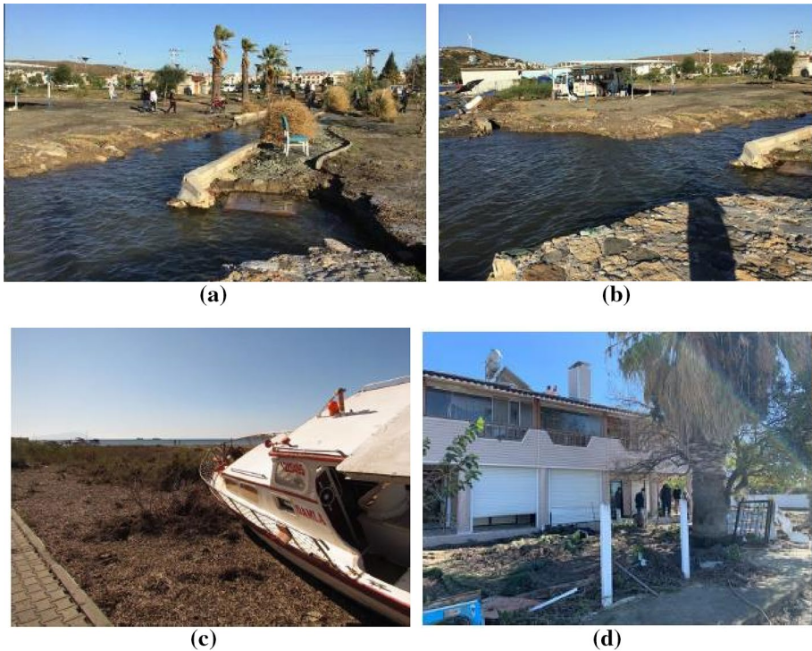
Fig. 45 a, b and c maximum inundation distance d maximum flow depth (METU 2020)
