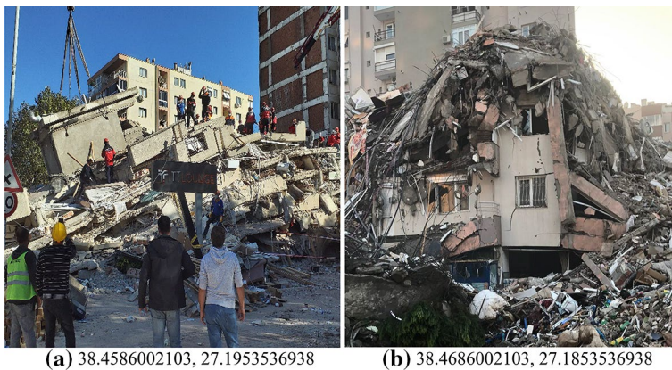
Fig. 29 Total collapse due to strong beam-weak column
