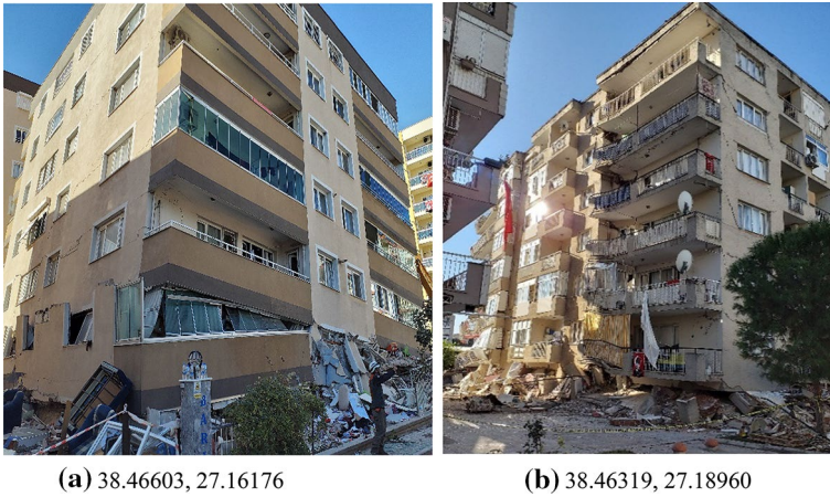
Fig. 32 Soft-story mechanism
