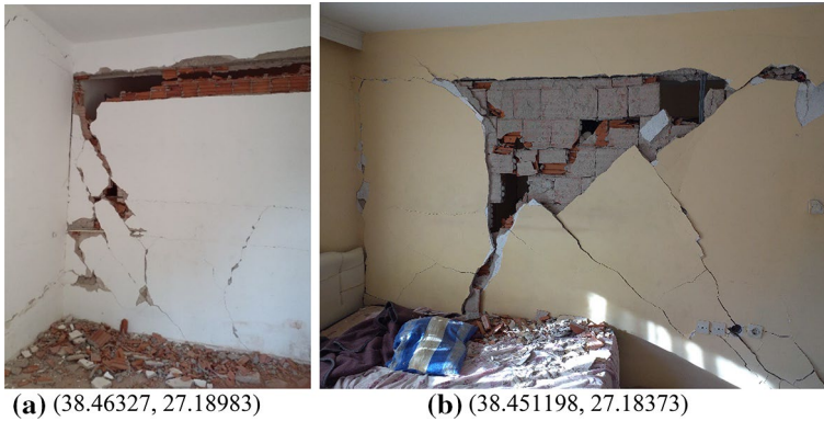
Fig. 37 Combined mechanism of infill walls
