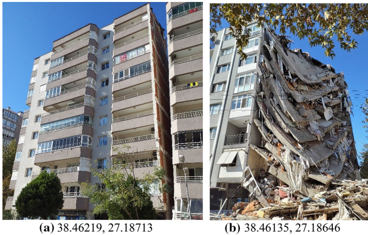
Fig. 28 Damages to adjacent buildings during the September 30, 2020, Aegean Sea earthquake
