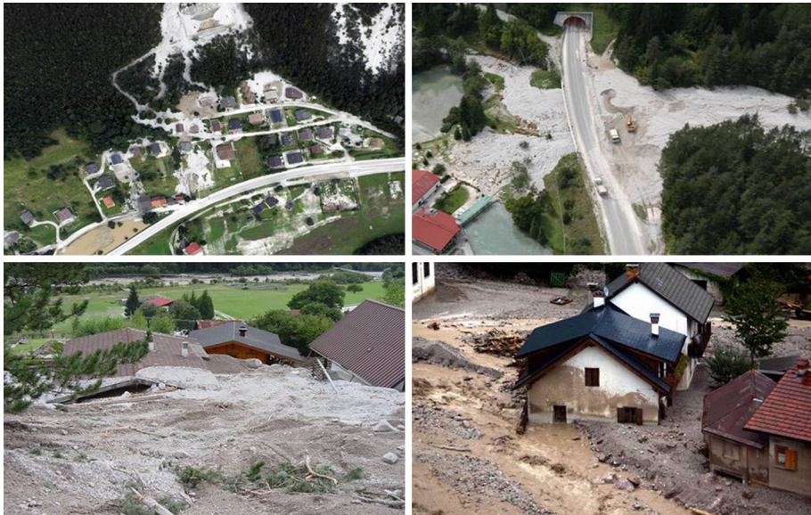
Fig. 2 Damage produced by debris flows and flash floods to infrastructure and buildings in the aftermath of the August 2003 event (source: Civil Protection, FVG Region, 2012)
