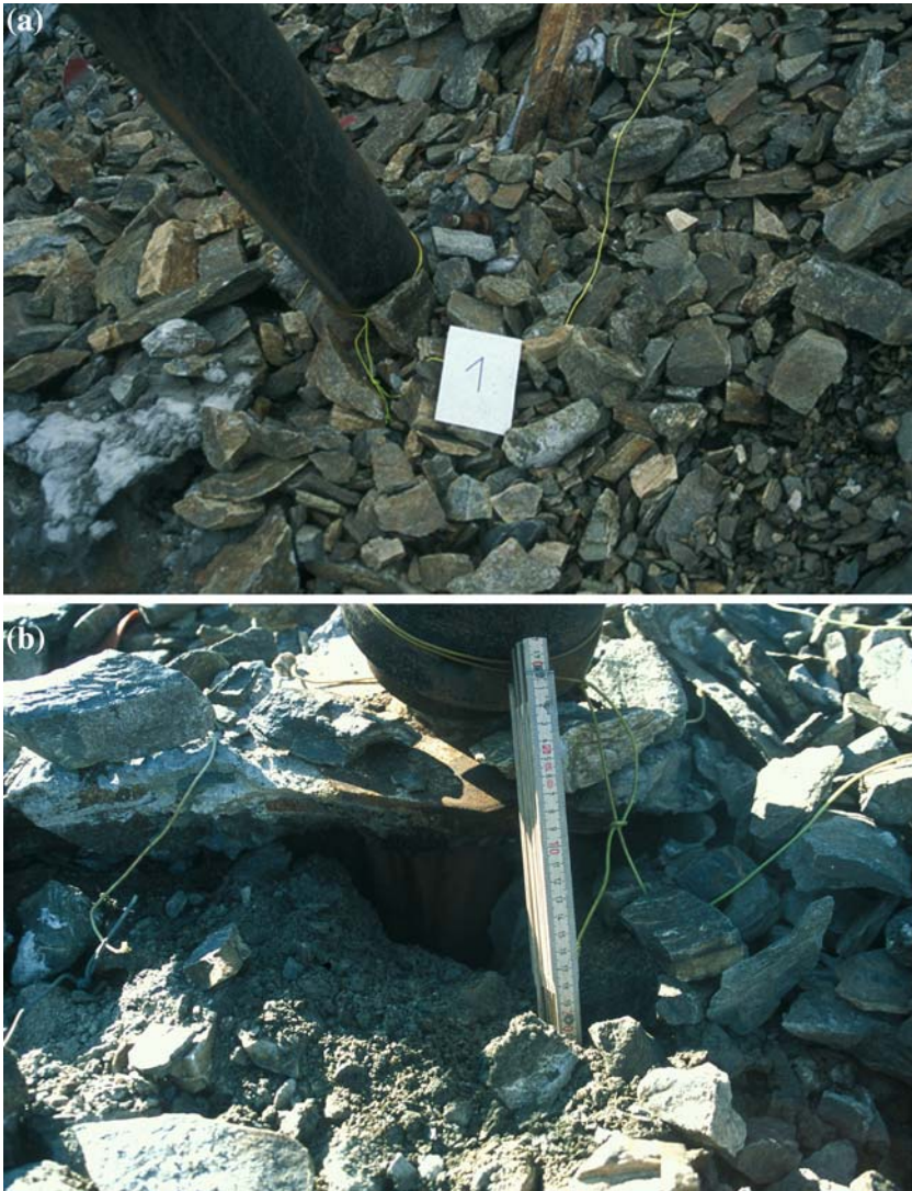
Figure 10. (a) A snow-bridge anchor (micropile) at Site 2 in 1997. (b) The same anchor in 2003 showing the denudation of the top of the anchor and surface erosion of the scree around the anchor head.
