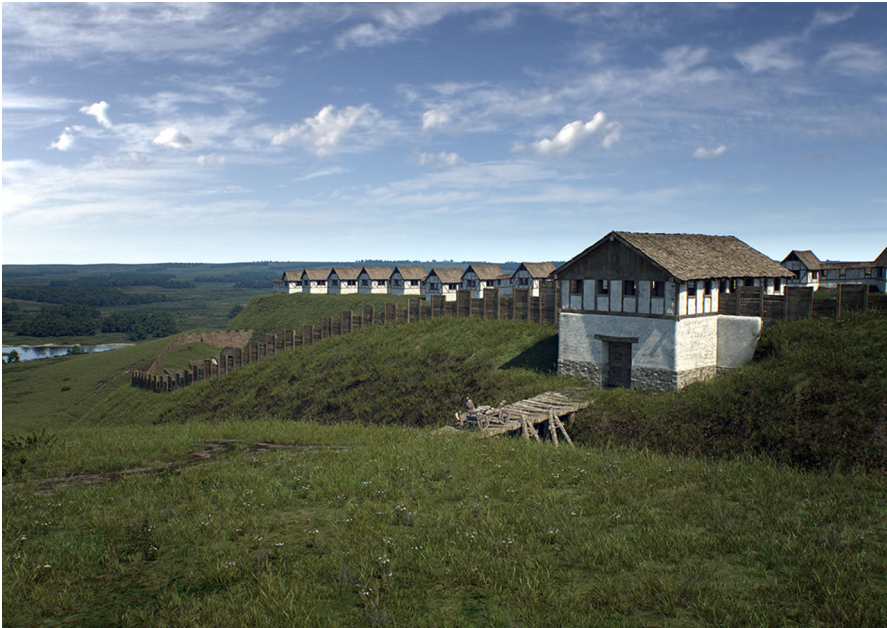
Fig. 3 Entrance gatehouse to the lower town of the Heuneburg, with mudbrick wall and towers of the acropolis in the background (after Krausse et al. 2016; design Faber Courtial; © Landesamt für Denkmalpflege im RP Stuttgart)
