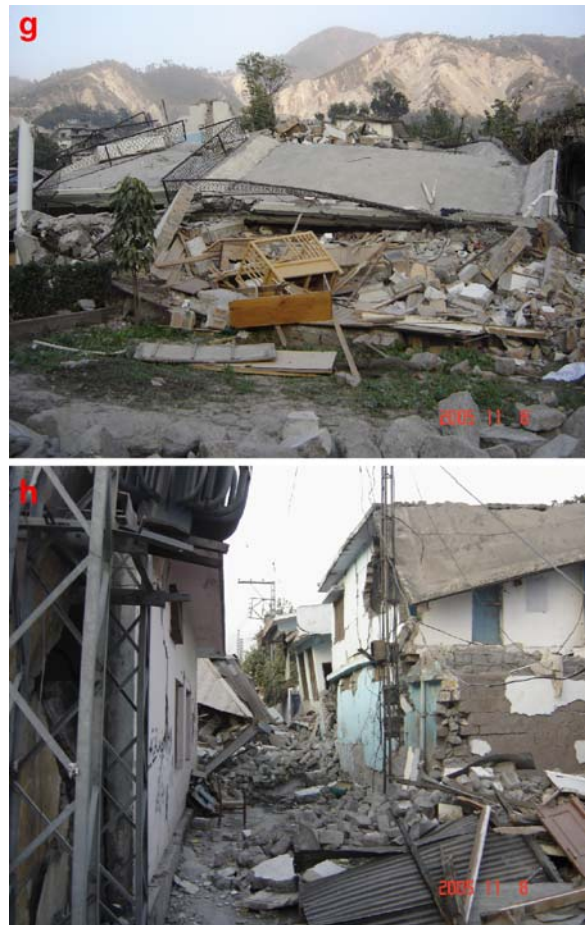
Fig. 7 Landslides (a–e; courtesy of National Engineering Services Pakistan) and destruction (f–h) in Muzaffarabad and Balakot
