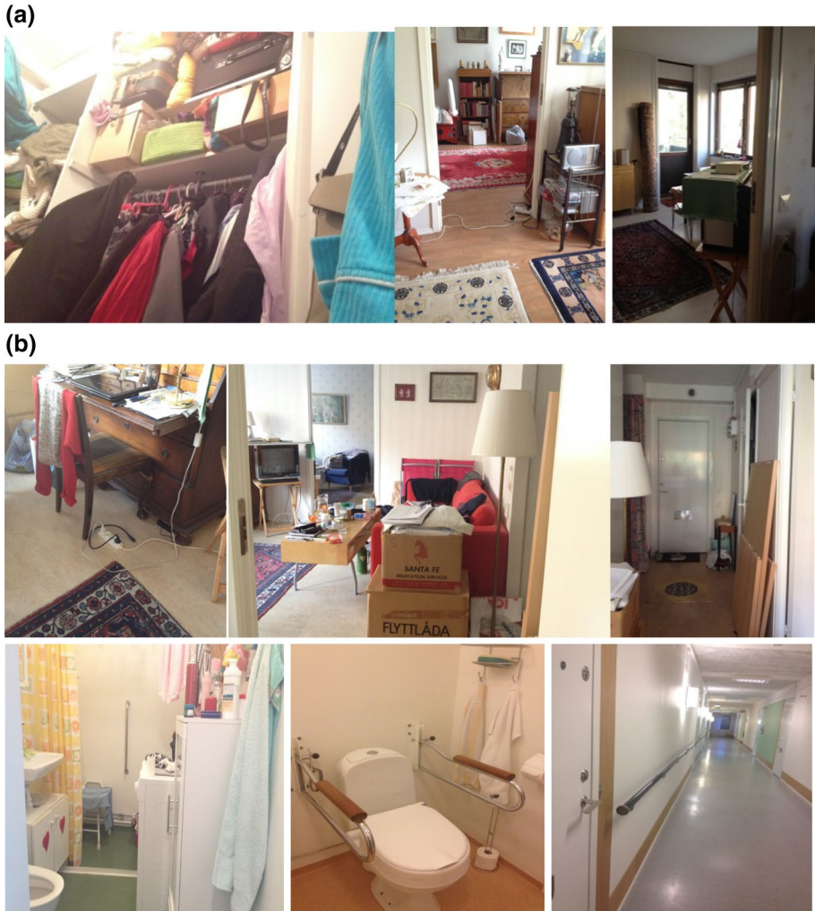
Fig. 4 a Hässelgården's senior housing—environmental features such as electrical cords, boxes and tables that promote accidents. Photographs: Bamzar (2014). b Features promoting safety: presence of handrails and grab bars in the bathroom and toilets and sufficient illumination in the corridor. Hässelgården's senior housing. Photographs: Bamzar (2014)
