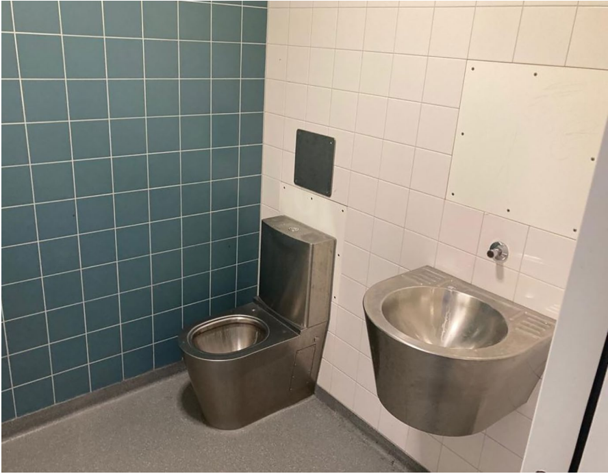
Fig. 10 Roberts bathroom before
