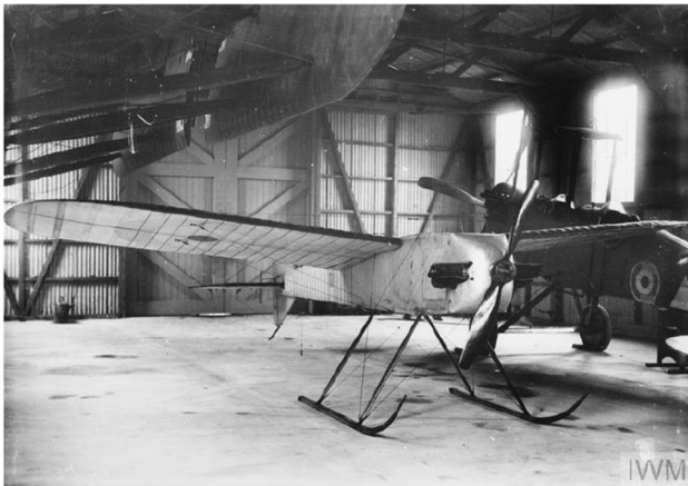
Fig. 1 Aerial Target, a British radio-controlled aircraft from the First World War ( https://www.iwm.org.uk/collections/item/object/205315299 )
