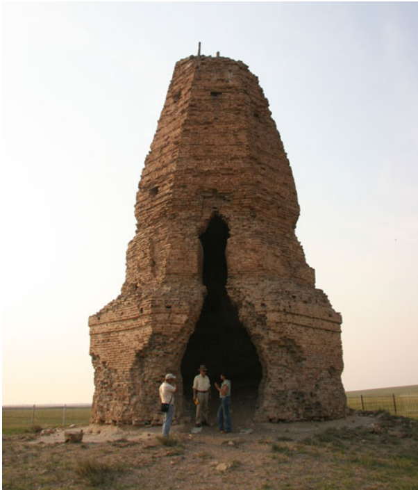
Fig. 4 Multistoried brick stupa at the Khitan Liao settlement of Kherlem Bars 1 (photograph by Amelia Yonan)
