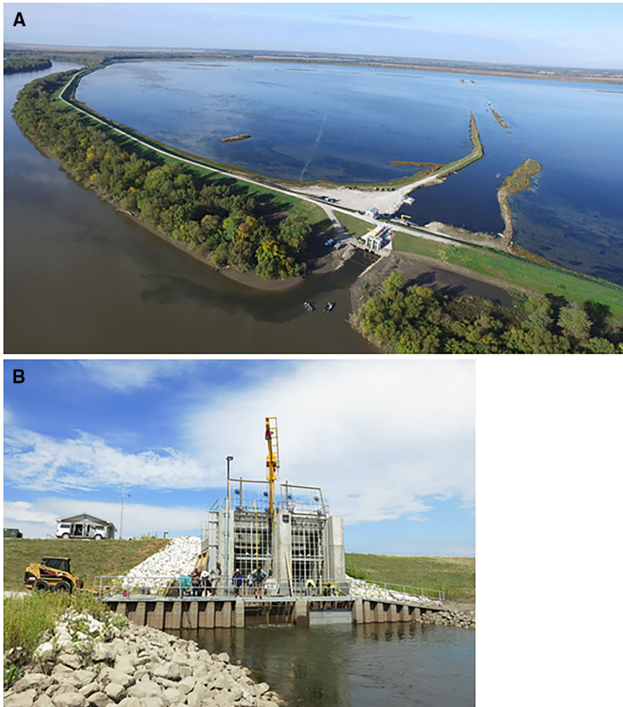
Fig. 5 A Emiquon Preserve ( right ) and Illinois River ( left ) on October 19, 2016. Clear water was being discharged from Emiquon into the Illinois River. Anglers in two boats are fishing in the discharge. The former agricultural drainage ditch, lined with trees and shrubs, extends into the distance at the right (Photo: D. Blodgett). B Looking from the Illinois River toward the gate structure in the Emiquon levee. The yellow crane on top of the structure is used to lift nets, other sampling devices, screens, and metal stop “logs” in and out of the gates. Stop logs
