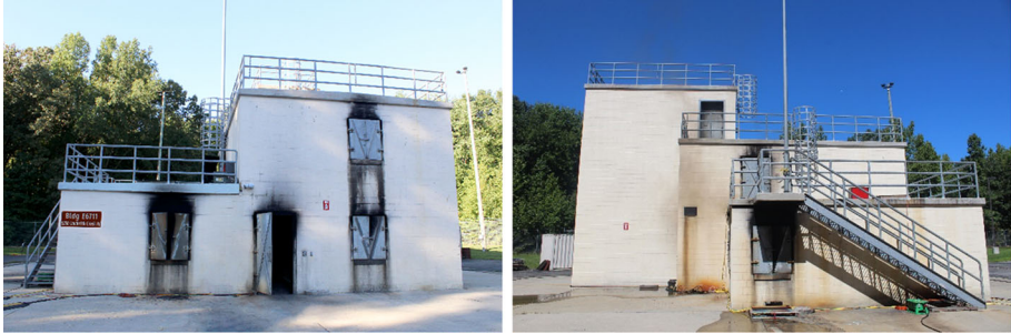
Figure 1. Multicompartment training structure at the Maryland Fire Rescue Institute. (Left) front view with burn room on the left and hallway in the middle. (Right) side view showing burn room, stairs to second floor landing above the burn room and three-storey stairwell.
