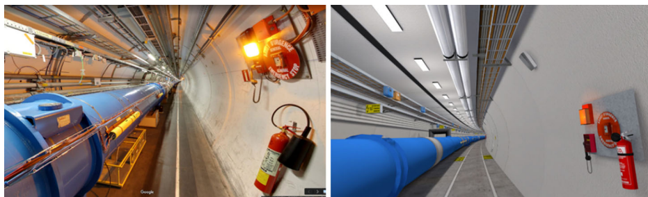
Figure 1. Actual tunnel accelerator configuration (of the Large Hadron Collider at CERN, taken from Google street view, retrieved in 2017, with a cross section of approximately 3 m) on the left versus virtual tunnel environment of the Future Circular Collider on the right, with a cross section of approximately 6 m.
