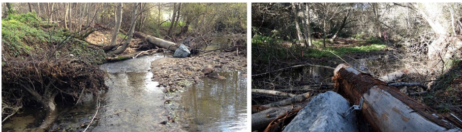
Fig. 2 Images of the woody structures positioned in the construction sites to regulate flow direction
