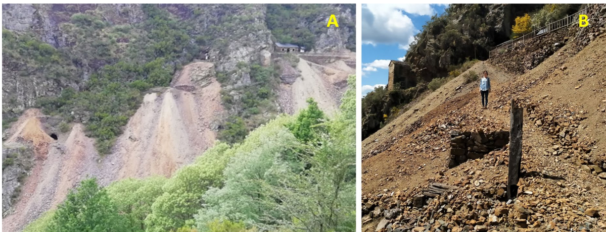
Fig. 1 Some galleries and the hosting quartzites above the spoil heaps of the Carmina mine (A); Details of the spoil heaps (B)
