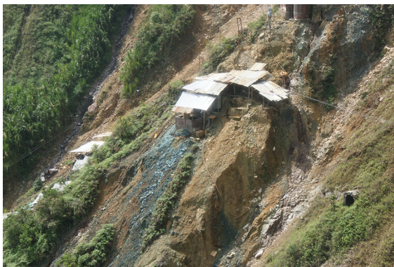
Fig. 3 A small entable near Marmato, Colombia, built on a precarious slope to process gold ore. Note the distinctive blue ferrocyanide staining from cyanide discharges from the mill. A small adit is visible in the right foreground
