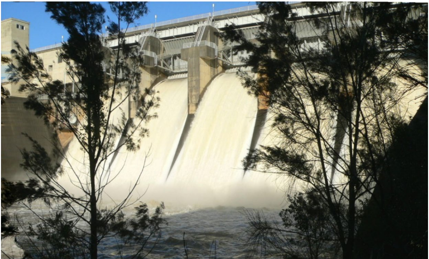
(B) North Pine Dam smooth spillway (Australia) in operation on 22 May 2009
