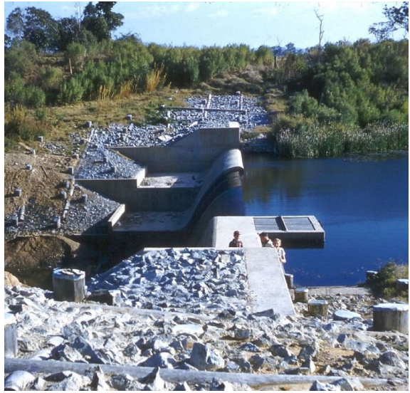
Fig. 3 In-stream weir on Wararba Creek weir near Caboolture (Australia) in the 1960s (Photographer Roy Dobson. Image courtesy of Moreton Bay Regional Council, reference number CLPC-P2299)
