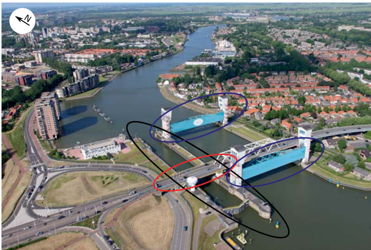
Fig. 1 The Algeira complex consisting of a lock (encircled in black), a bascule bridge (encircled in red), and two storm surge barriers (encircled in blue) [ https://beeldbank.rws.nl , Rijkswaterstaat / Joop van Houdt]
