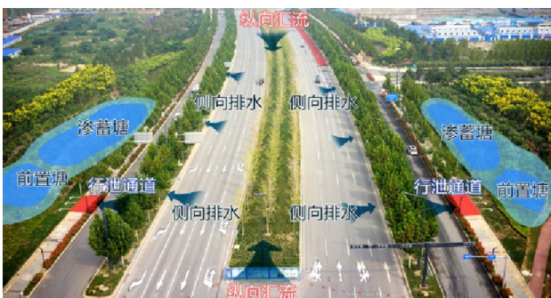
Fig. 13 Photos showing the of integrated drainage system within Qinhuang Avenue
