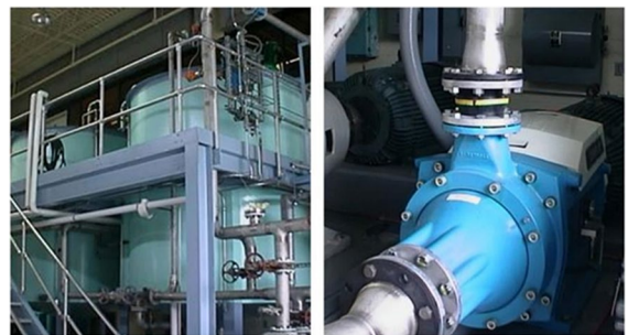
Fig. 1 UMaine thermo-mechanical refiner at process development center (PDC)
