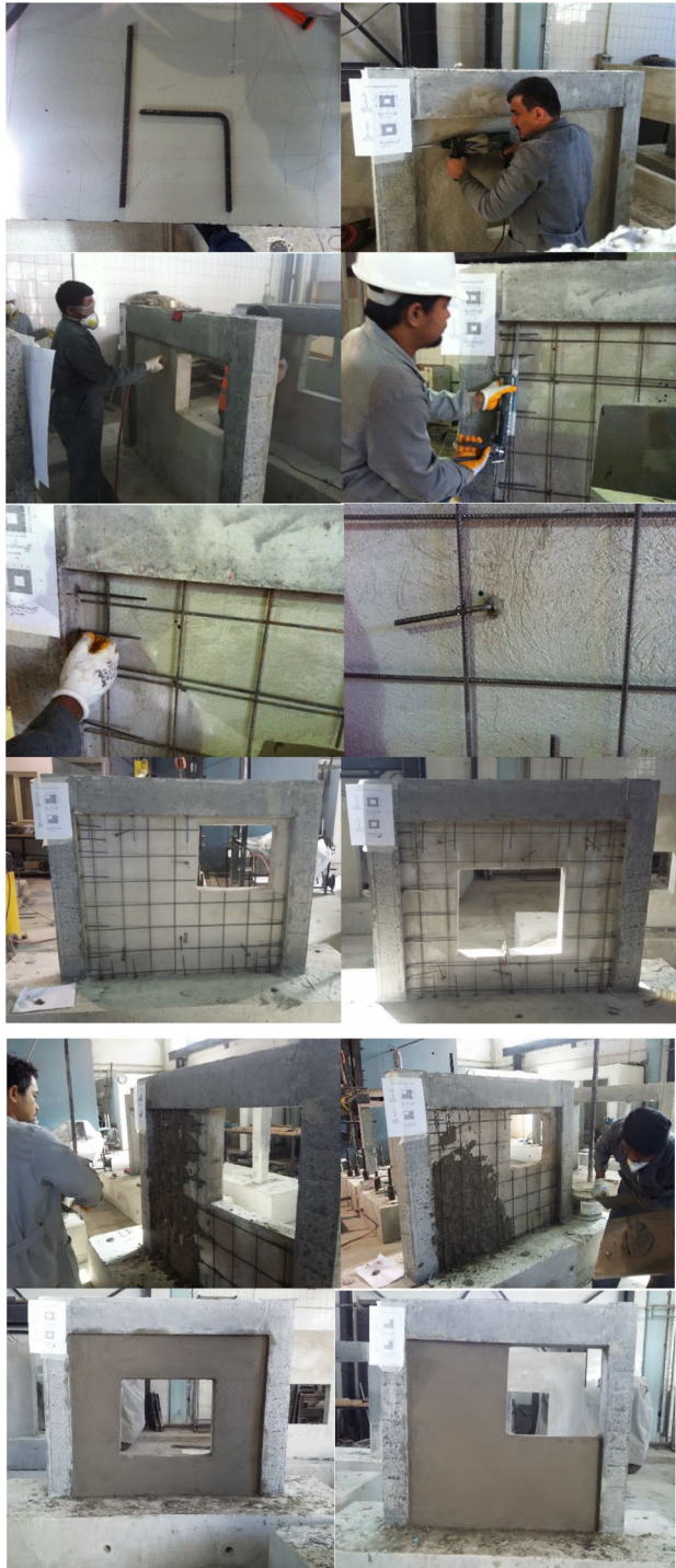
Fig. 4 Strengthening application step photos of specimens
