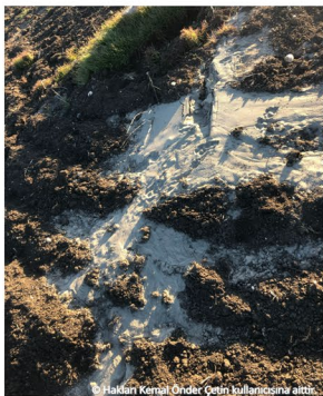
Sand boils at Lat:37.337105°N, Long:37.045719°E
