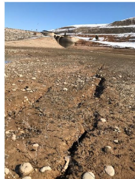
Lateral spreading at Lat:38.34652°N, Long: 38.0593°E
