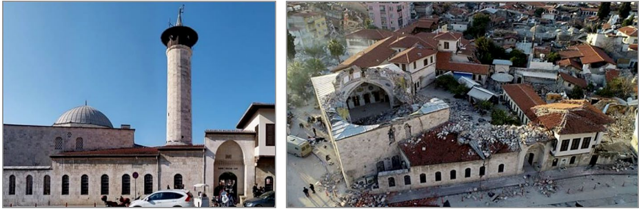
Fig. 21 Habibi Neccar Mosque, Antakya, Hatay, before (left) and after (right) the Kahramanmaraş earthquakes
