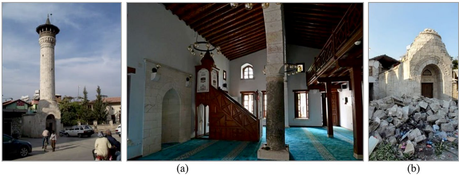
Fig. 22 Sarimiye Mosque, Antakya, Hatay, before (a) and after (b) the Kahramanmaraş earthquakes
