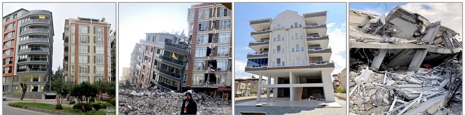
(a) Building 1, before (left) and after (right) earthquakes (b) Building 2, before (left) and after (right) earthquakes
