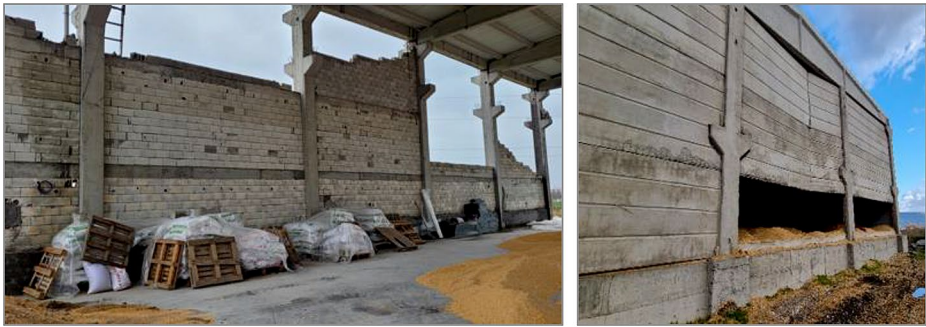
Fig. 20 Examples of large-span walls exceeding the maximum unsupported wall length on the walls (left) and out-of-plane tipping damage on the precast wall panels (right)
