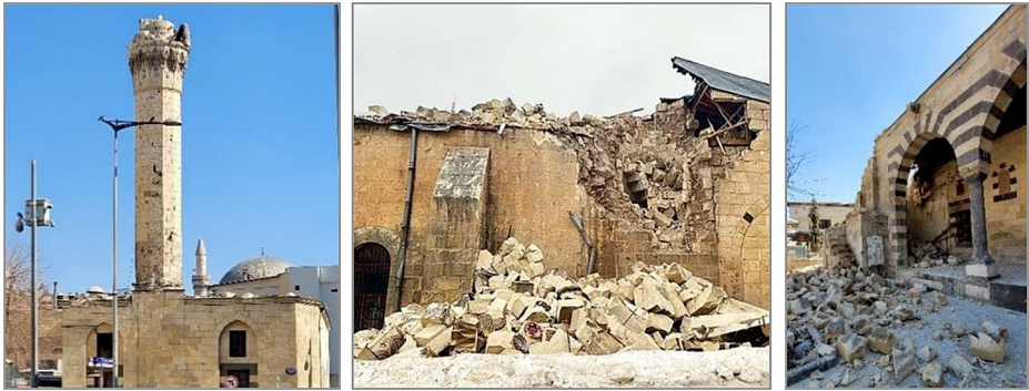
Fig. 27 Examples of damage to minarets
